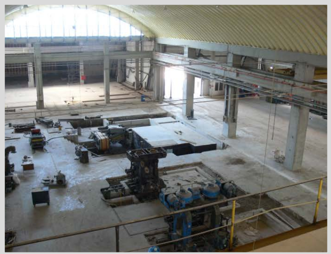
Makine temelleri / Machine foundations
