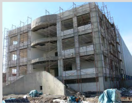
İdari Bina Administrative Building
